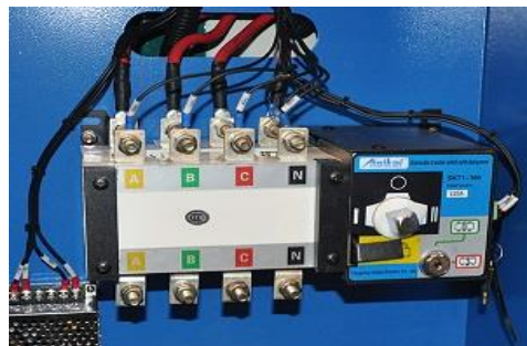
ATS Automatic Transfer Switch
